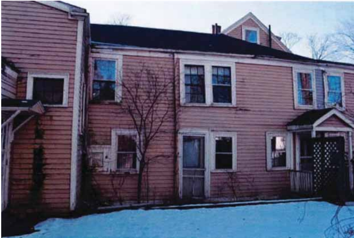
Nathaniel Allen House, Description of Rehabilitation
