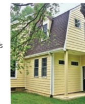
◀ A GARAGE ADU makes use of an attached or detached garage by converting the space into a residence. Other options involve adding a second-story ADU above a garage or building a new structure for both people and cars.
