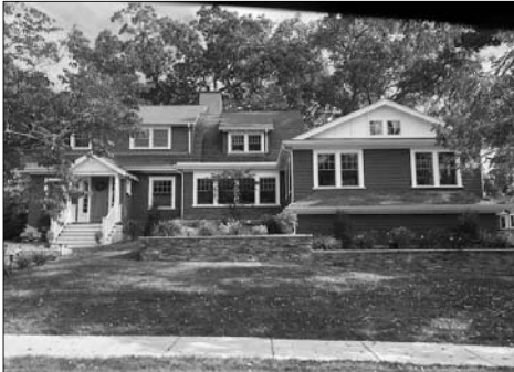
DESCRIPTION HERE- the garage is forward of the front façade and is designed in this way because of limitations with the rear lot setback. This could not be done with the garage ordinance as written
