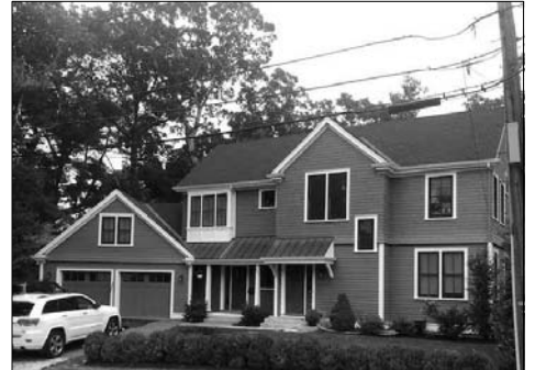
DESCRIPTION HERE- the garage is forward of the front façade by 4' due the rear lot setback
