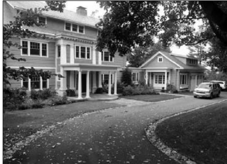
DESCRIPTION HERE- the garage is forward of the front façade and is designed in this way because of limitations with the slope rear lot setback. This could not be done with the garage ordinance as written
