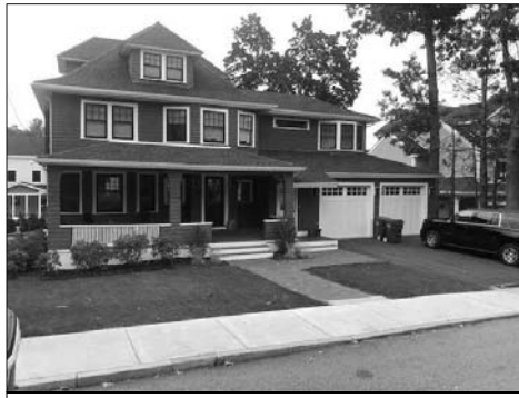
DESCRIPTION HERE- the garage is forward of the front façade by 4' due the rear lot set back and also is too wide
