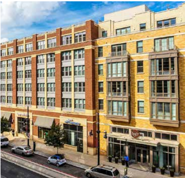
Figure 6.2.9 Appearance of Two Buildings
