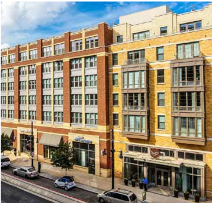
Figure 5.1.11 (a) Appearance of Two Buildings
