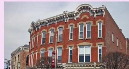
Shape the roofs of buildings
