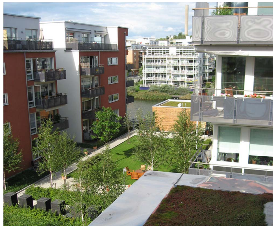
Example new construction in the Stockholm eco-district of Hammarby Sjöstad integrate sustainable design features throughout, including the green roofs and pocket parks seen here as well as in the hidden stormwater, heating, electrical, and waste managements systems that are integrated throughout the development.
