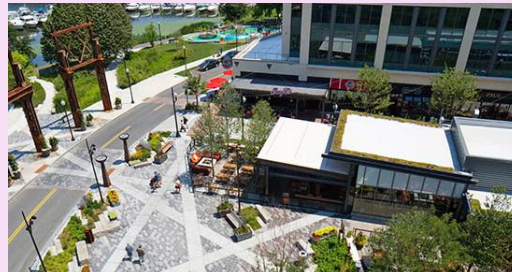
Design public open space as an extension of the streetscape and maximize comfort and visual access*
